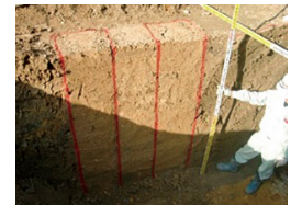
遮水壁断面確認
