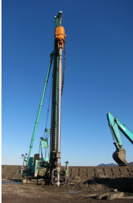
DCS掘削機全景
